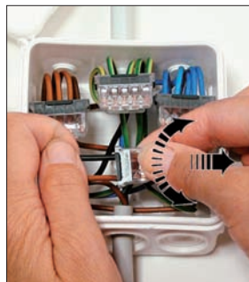
Releasing the wire through rotation and removal
